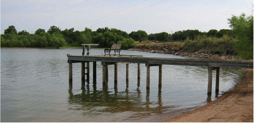
This is an example of a fixed dock supported by pilings.
