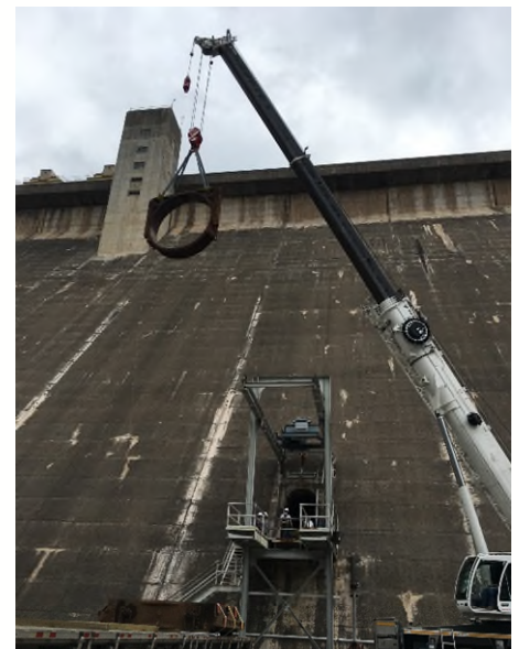
Mansfield Dam rehabilitation project, April 2019.
