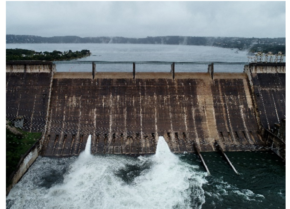
Mansfield Dam during flood operations in October 2018.
