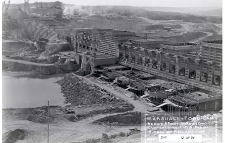
Mansfield Dam construction, 1938. (LCRA Archives W00170)
