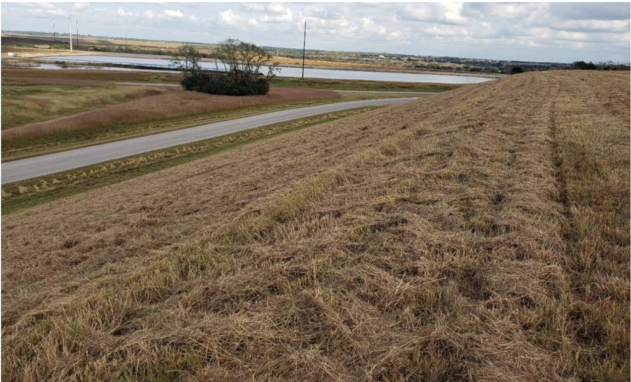
PHOTO 3 – View of Cell 1 North Embankment Slope during follow-up inspection (12-02-2021)
