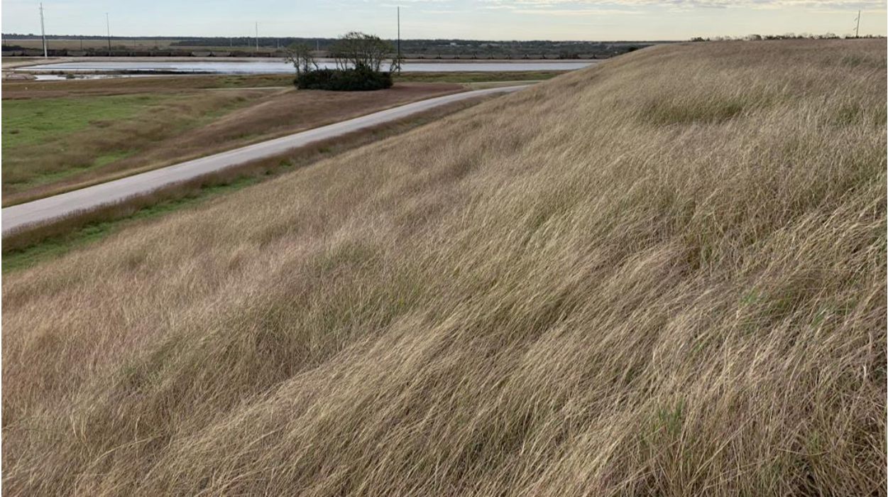
PHOTO 2 – View of Cell 1 North Embankment Slope during initial inspection (11-18-2021)
