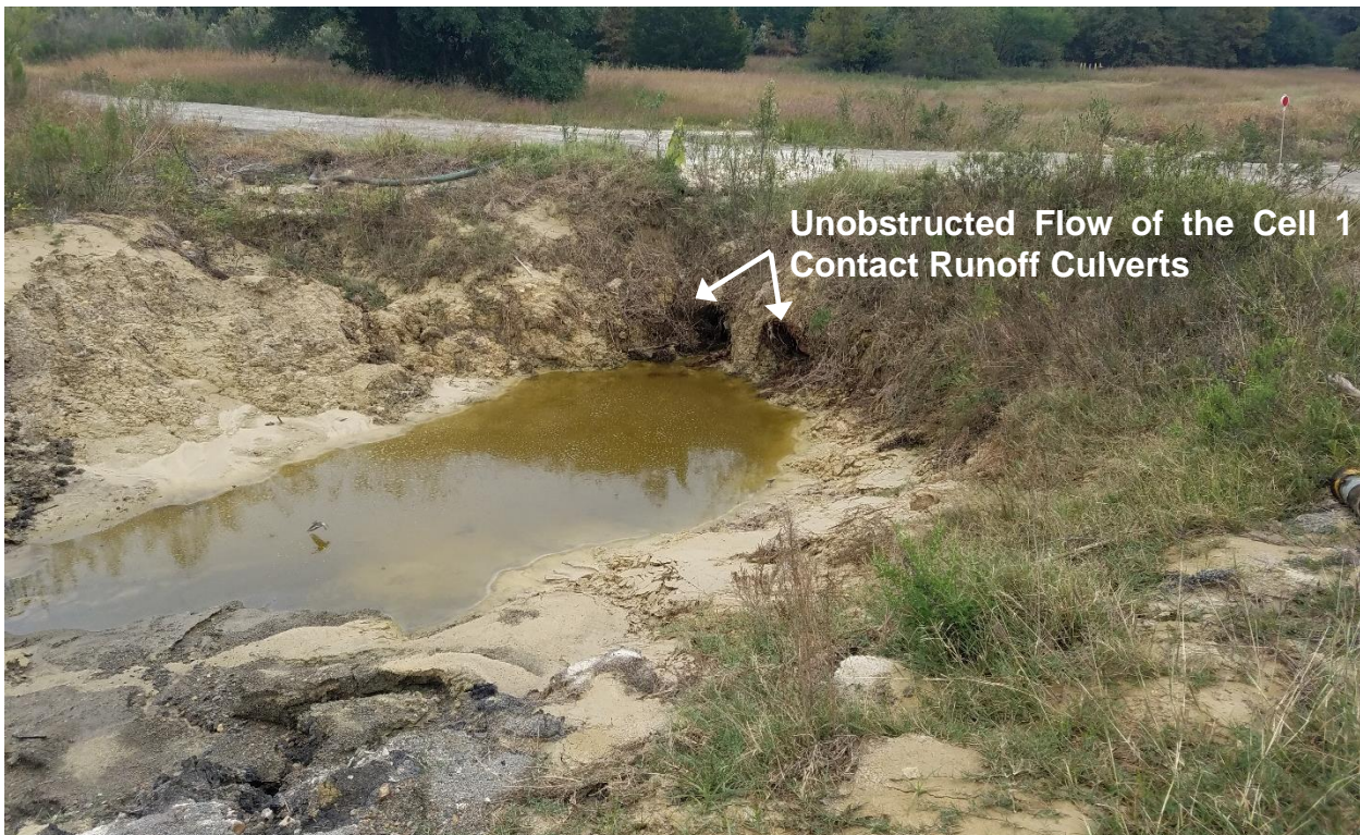
PHOTO 2 – View of unblocked inlets for Cell 1 stormwater channel culverts looking South (11-07-2019)
