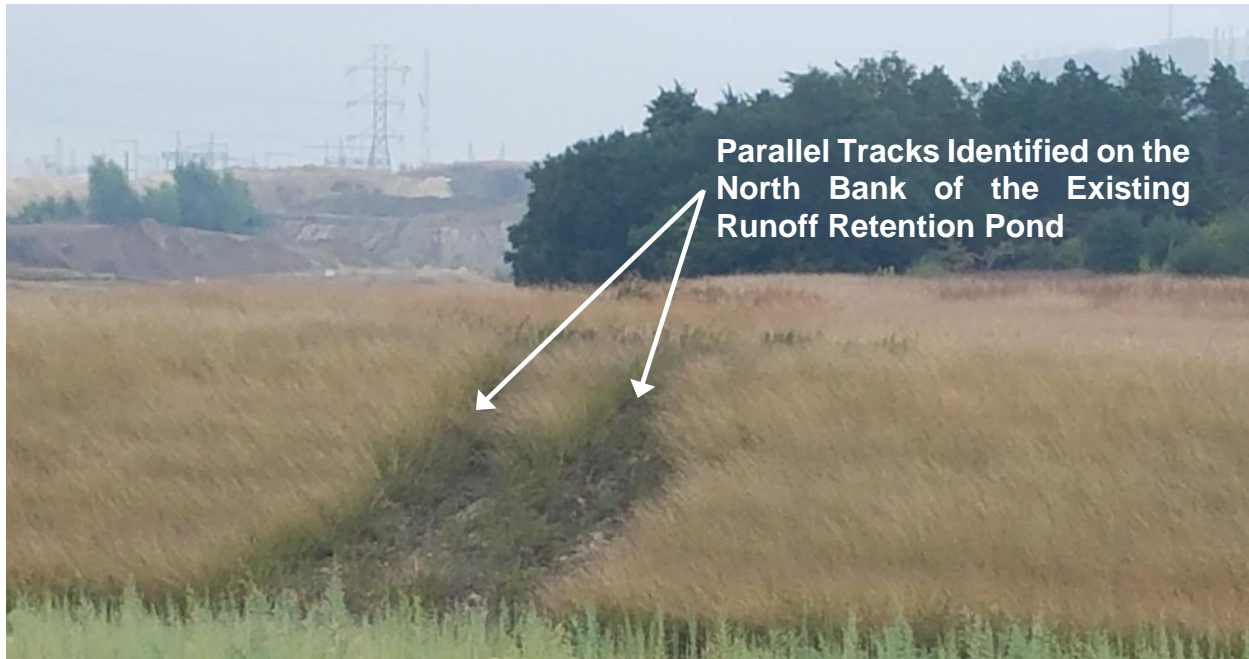
PHOTO 1 – View of vegetative discontinuity identified on the Cell 1 Existing Runoff Retention Pond North cut bank (11-07-2019)
