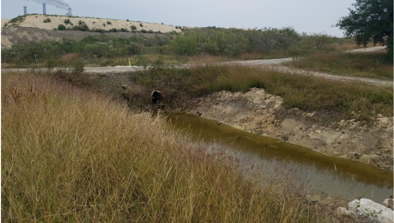
PHOTO 3 – View of unblocked Cell 1 stormwater channel culvert outlets looking North (11-07-2019)
