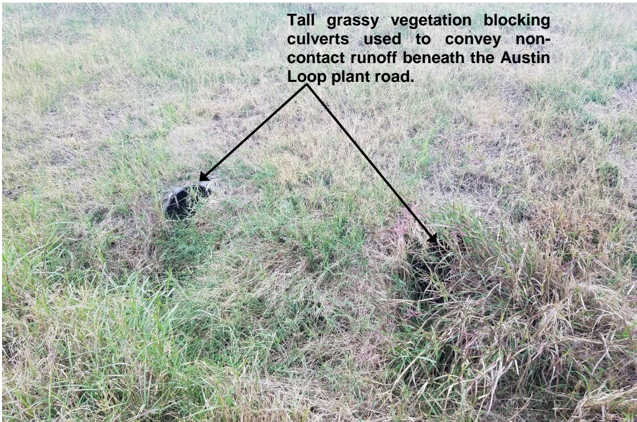
PHOTO 4 – View of grassy vegetation blocking culverts northeast of Cell 1 (11-7-2019)
