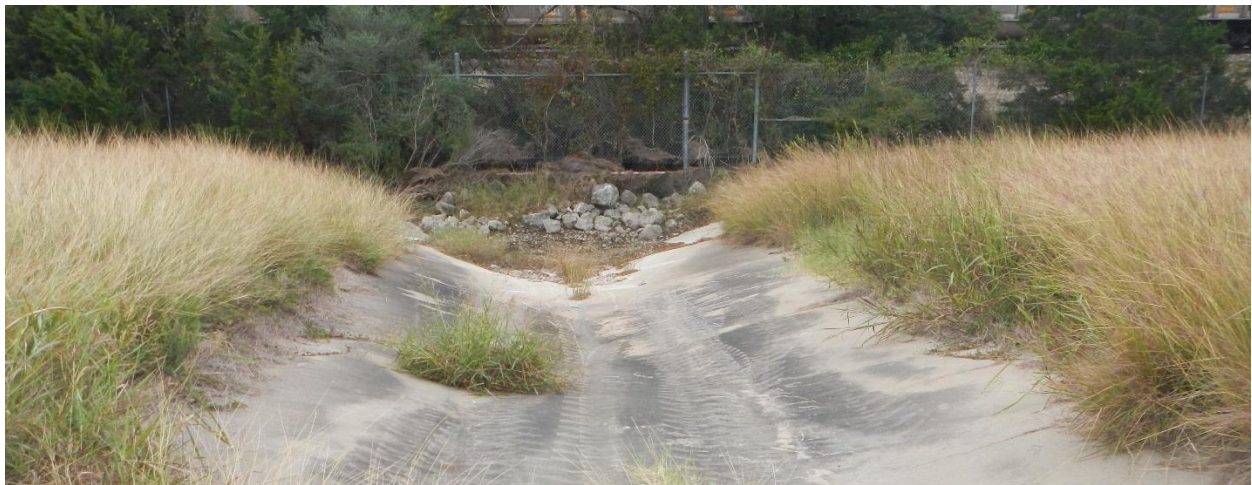
PHOTO 4 – View of cleared CBL Runoff Pond Spillway Looking South (11-18-2017)
