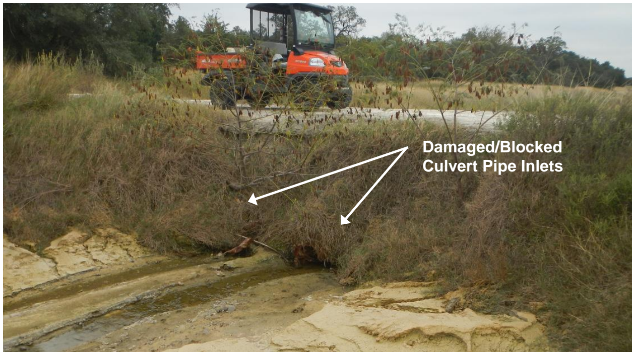
PHOTO 2 – View of Cell 1 Stormwater Channel culverts looking Southeast (11-8-2017)
