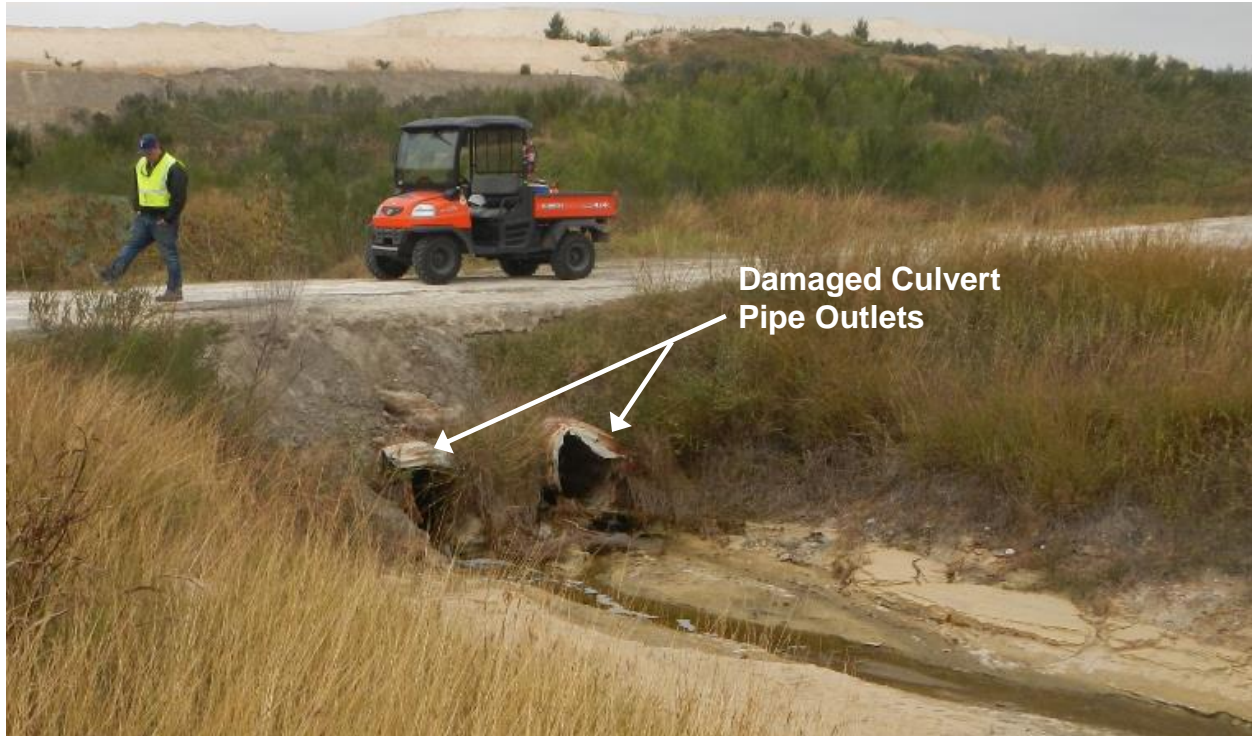
PHOTO 3 – View of Cell 1 stormwater channel culverts looking Northeast (11-8-2017)
