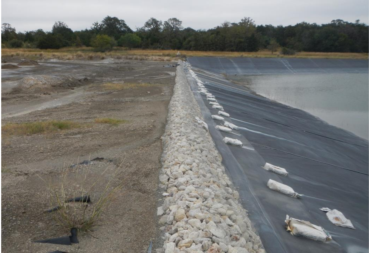
PHOTO 5 – View of repaired Subcell 2D Pond North Slope Rock Silt Berm (11-8-2017)
