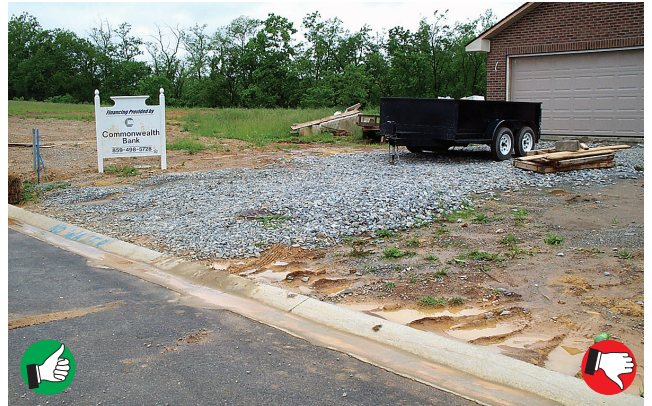
Rock sizing and placement look OK for a residential site, and very little mud appears on the pavement. The pad is a little thin, however, and it looks like some drivers are not using it—note track marks near curb. Adjacent soil areas need seed and mulch.
