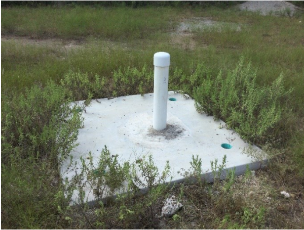
S-1: Water Well (Capped)
