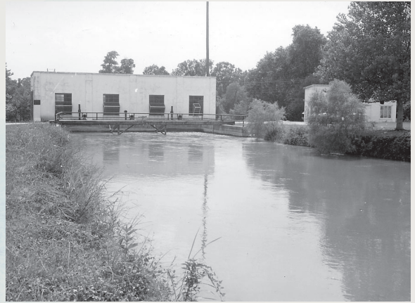
Canal and 1949 pump plant
