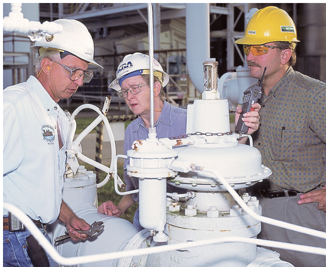
Employees at LCRA's Sim Gideon Power Plant conduct thorough safety inspections at the facility every quarter.
