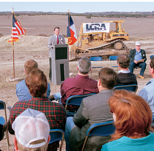
LCRA breaks ground on a reservoir and water treatment plant in Lometa, one of many projects to provide communities with reliable water and wastewater utilities.
