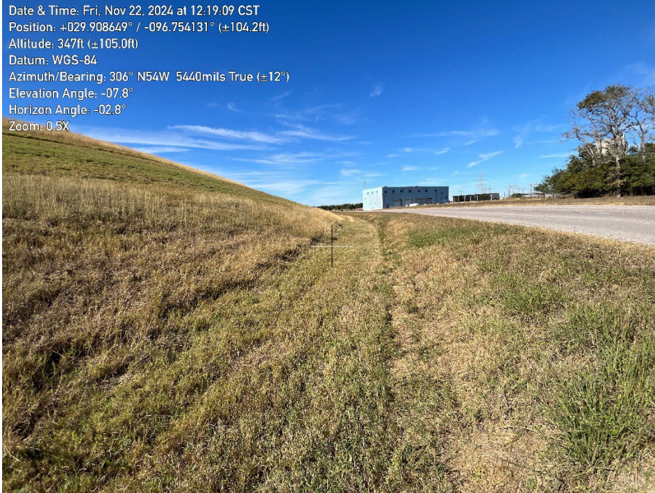
Photo 1 – Cell 1 North Embankment, Facing Northwest
