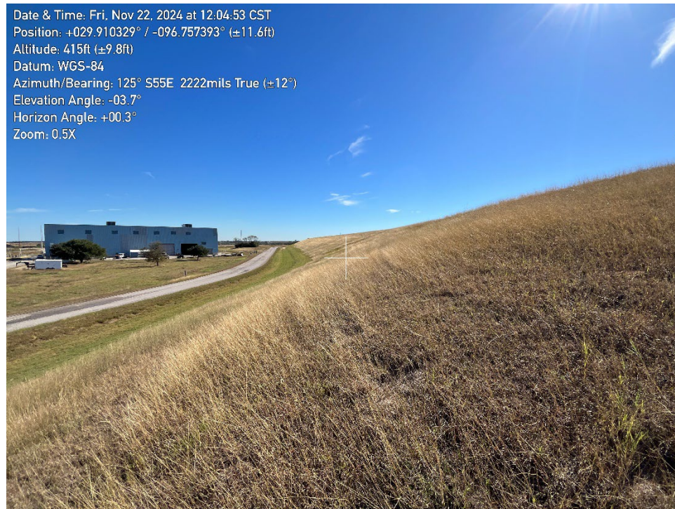
Photo 4 – Cell 1 North Embankment, Facing Southeast
