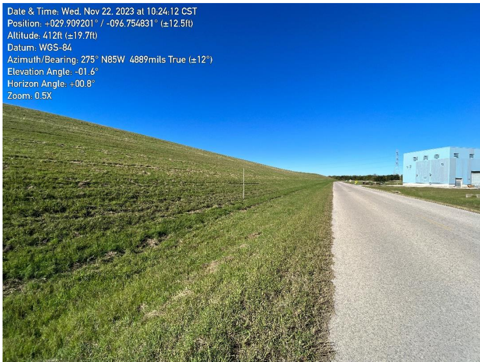
Photo 1 – Cell 1 North Embankment, Facing West
