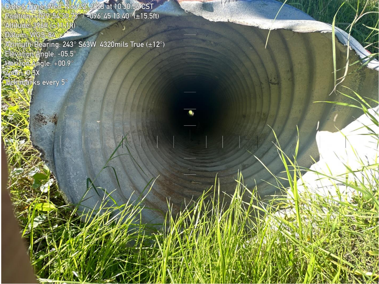
Photo 3 – Non-Contact Water Drainage Culvert at Northeast Corner of Cell 1, Facing Southwest
