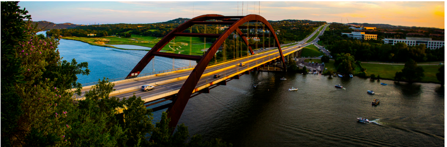
Loop 360 overlook and Pennybacker Bridge over Lake Austin
