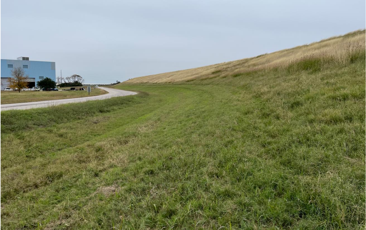
PHOTO 1 – View of Cell 1 North Embankment Looking East (12-01-2022)
