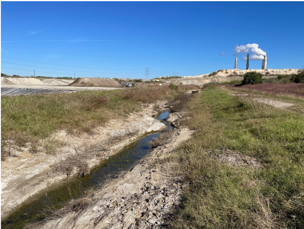
Photo 4. Existing runoff channel in project area
