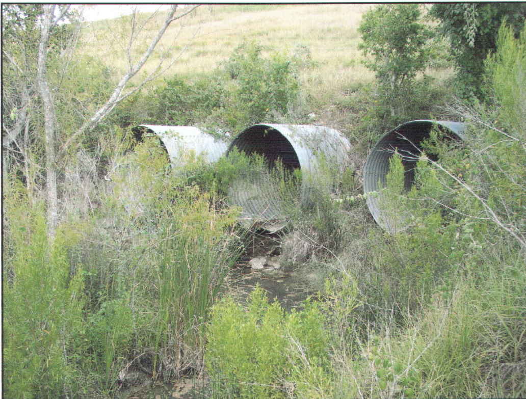
PHOTO 6: RAIL LINE CULVERT WITH WETLAND VEGETATION
