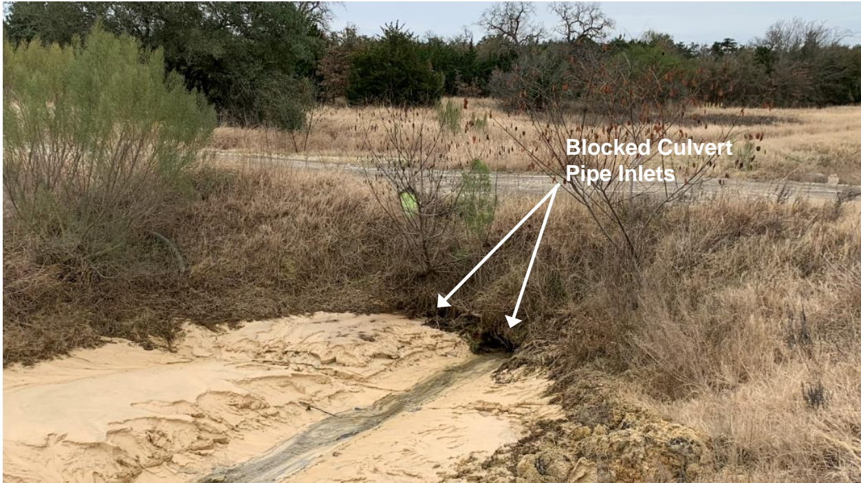
PHOTO 5 – View of Cell 1 Stormwater Channel culverts looking Southeast (12-12-2018)
