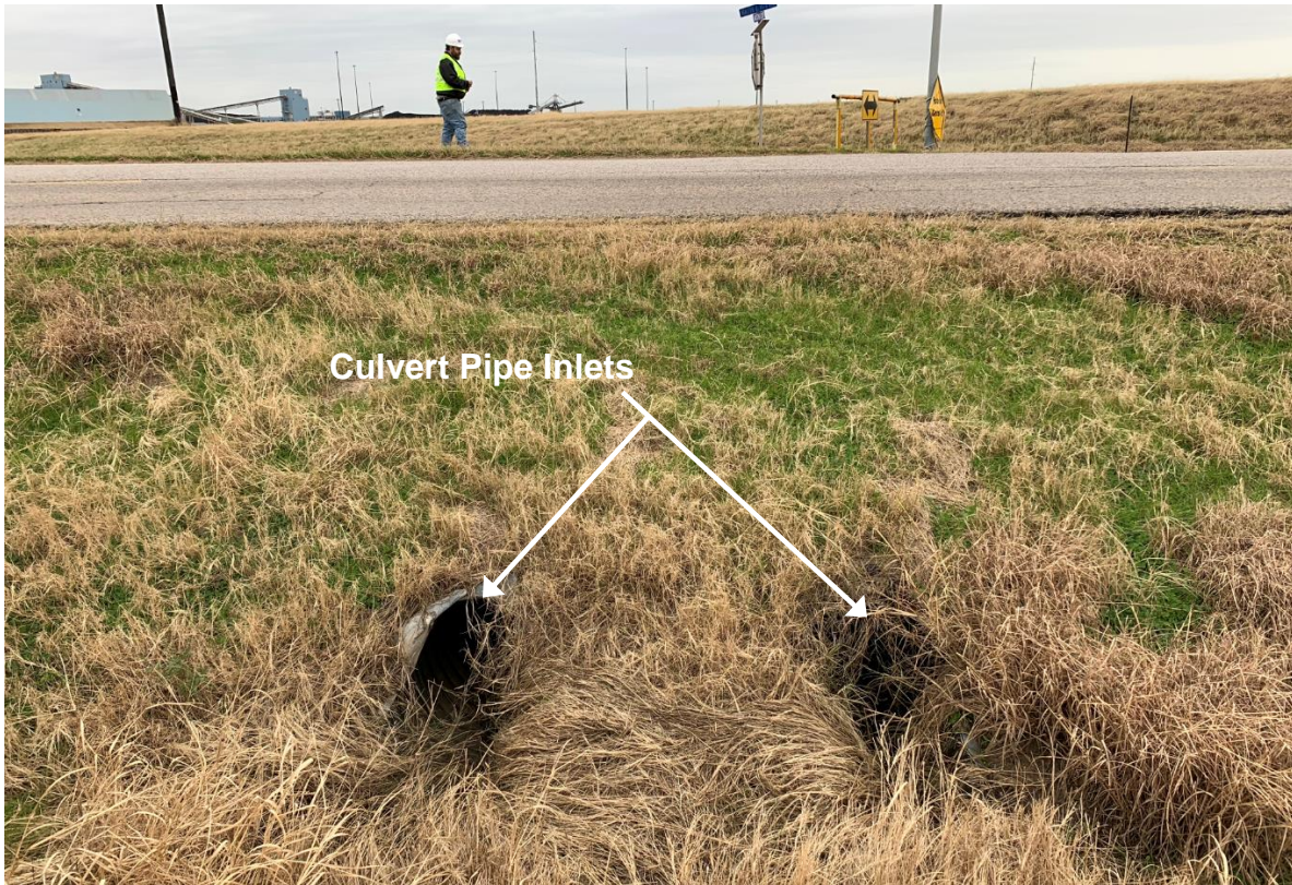
PHOTO 3 – View of repaired North Embankment culverts looking Northeast (12-12-2018)
