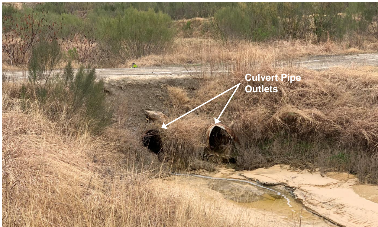
PHOTO 4 – View of repaired Cell 1 stormwater channel culverts looking Northeast (12-12-2018)
