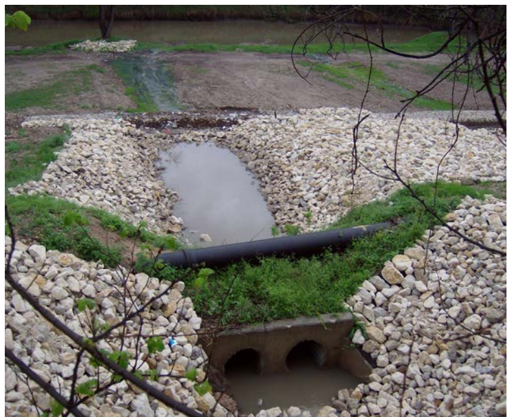
Gabion filter dam installed to capture pollutants during a rainfall runoff event in the Brady Creek watershed.
