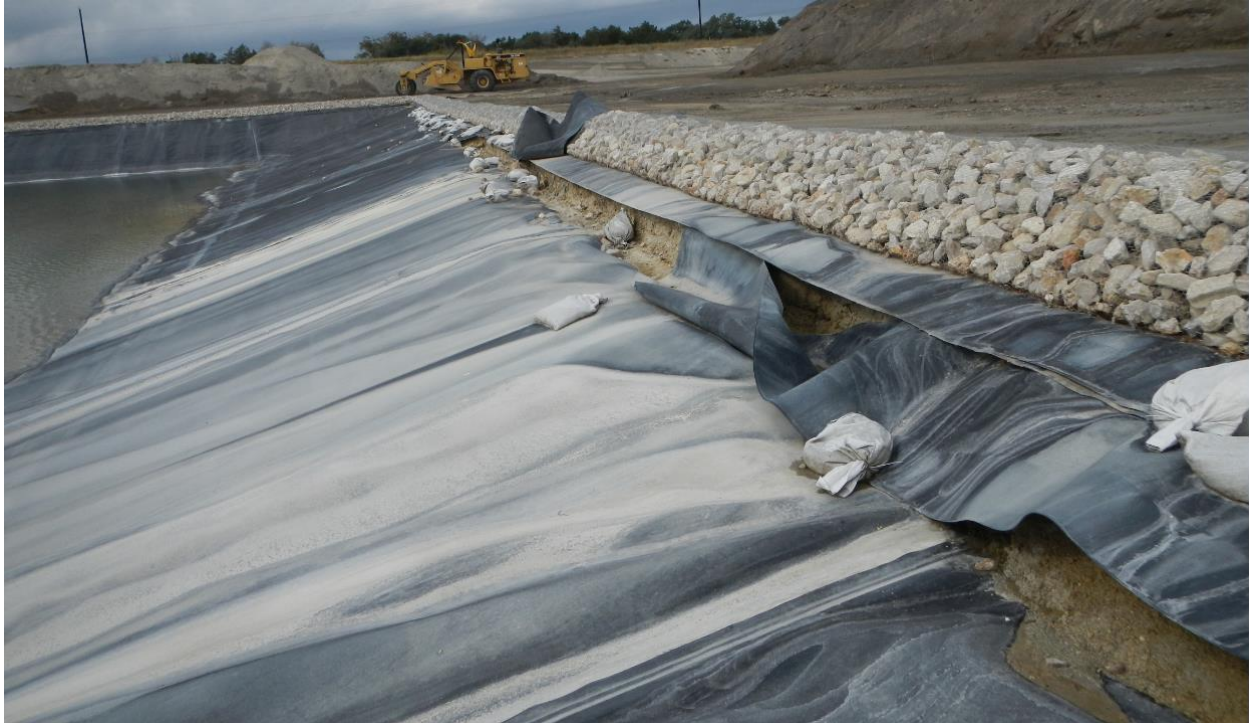
PHOTO 3 – View of Subcell 2D Pond North Slope Rock Silt Berm (11-18-2016)
