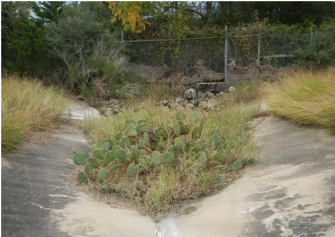
PHOTO 2 – View CBL Runoff Pond Spillway Looking South (11-18-2016)
