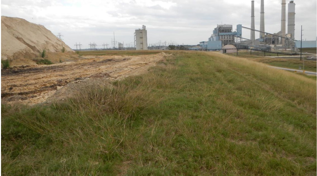
PHOTO 1 – View of East Embankment from Crest Looking North (11-18-2016)
