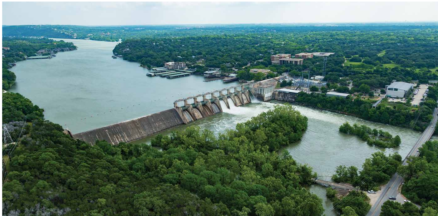
Tom Miller Dam at Lake Austin
