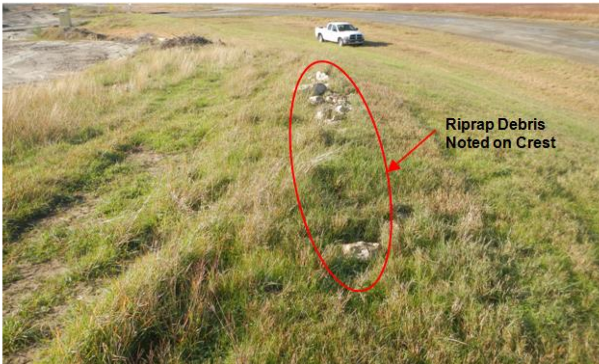
PHOTO 2 – View of West Embankment from Crest Looking South (12-09-2015)
