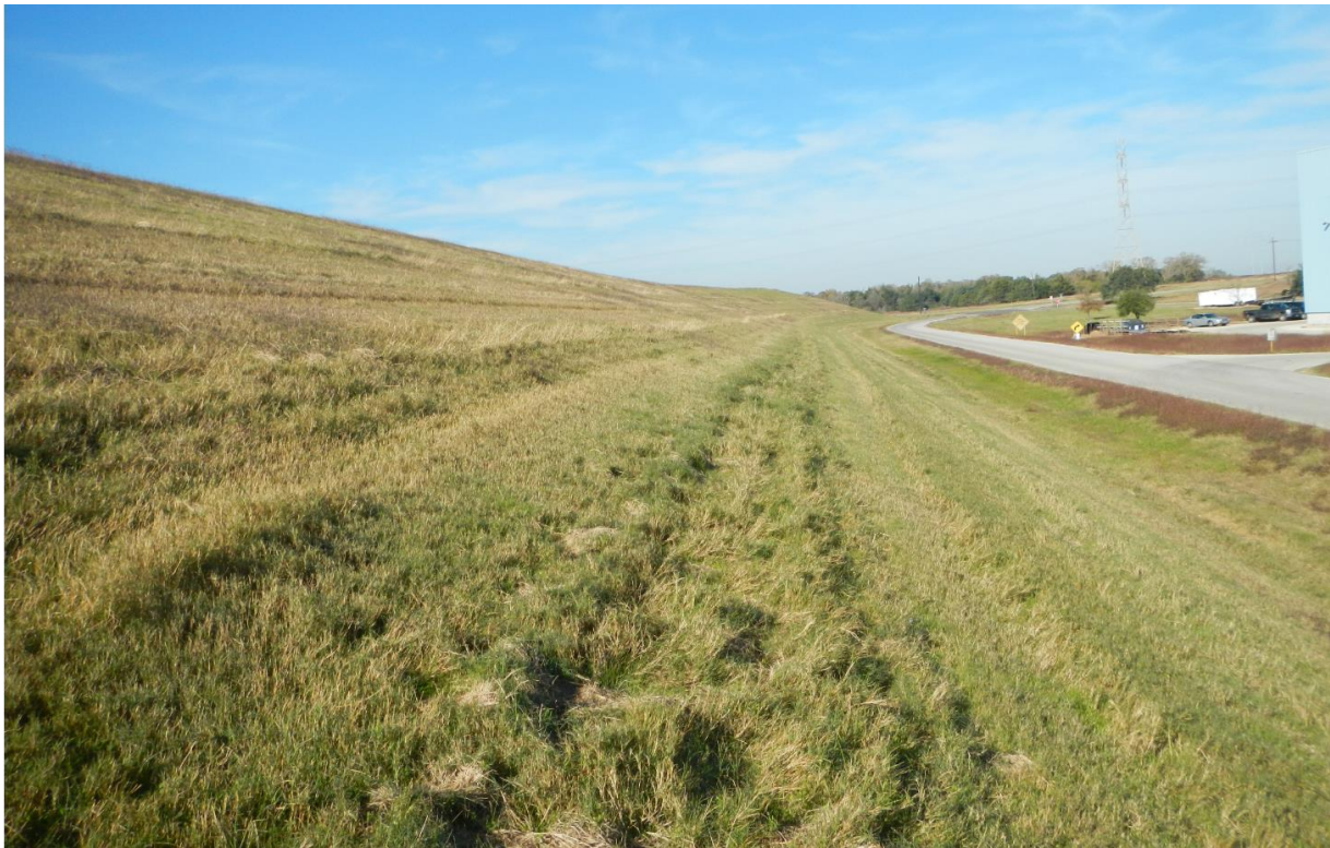
PHOTO 4 – View of North Embankment from Toe Looking West (12-09-2015)
