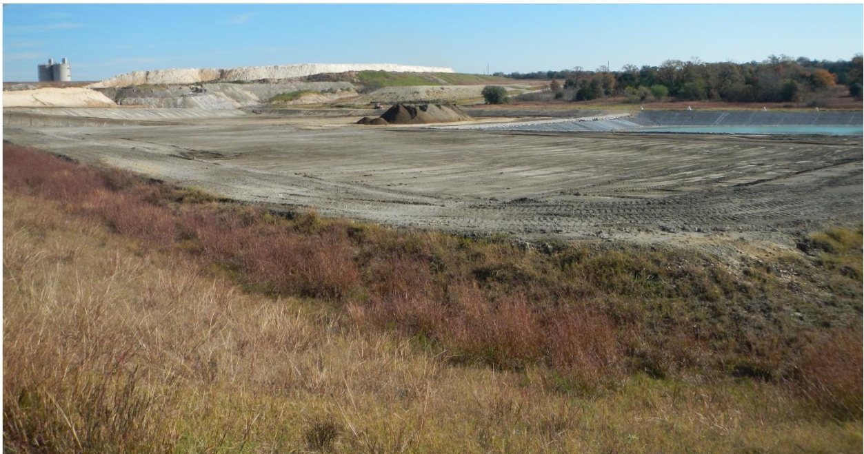
PHOTO 12 – View of CBL from Southwest Corner of Subcell 2D Storage Area (12-09-2015)
