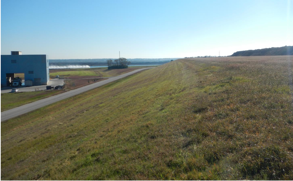
PHOTO 3 – View of North Embankment from Crest Looking East (12-09-2015)
