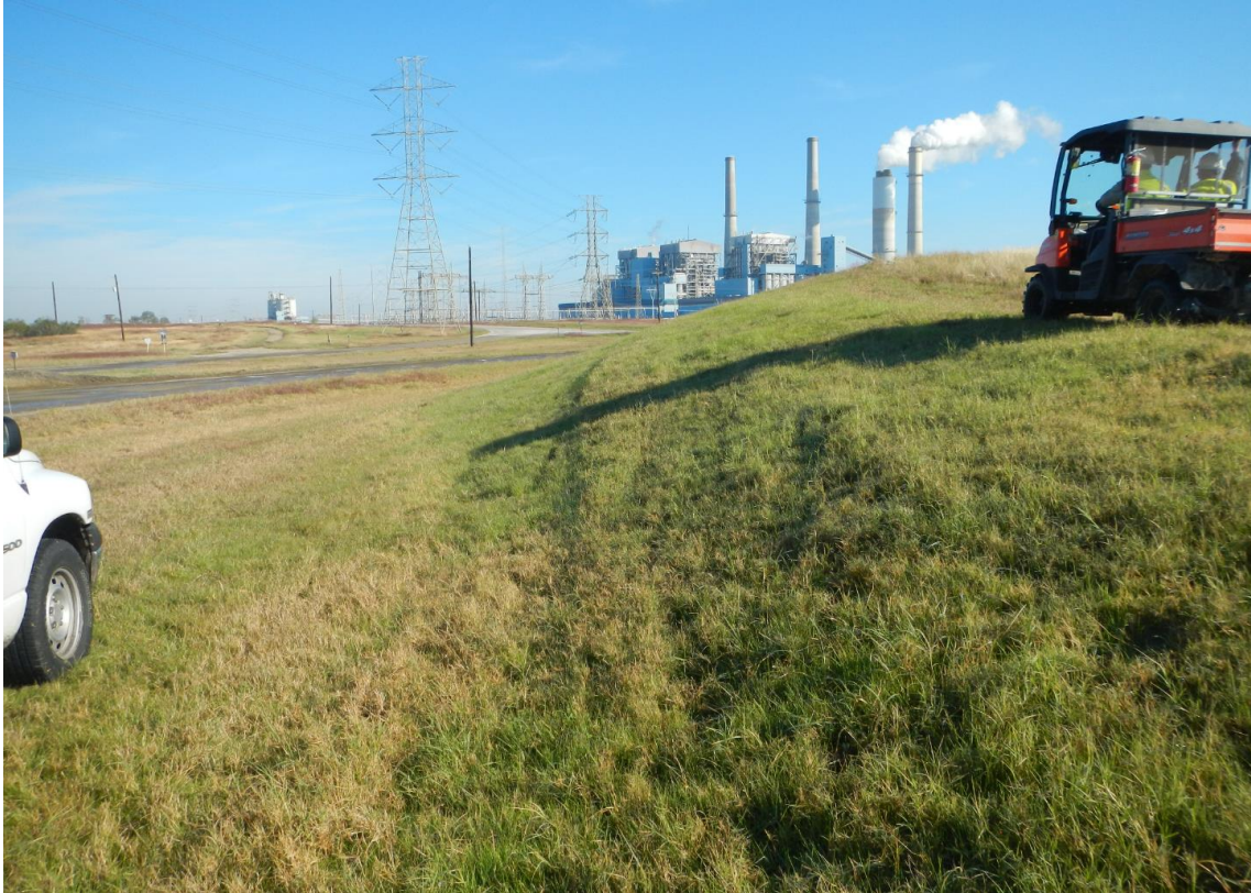
PHOTO 1 – View of West Embankment from Toe Looking North (12-09-2015)
