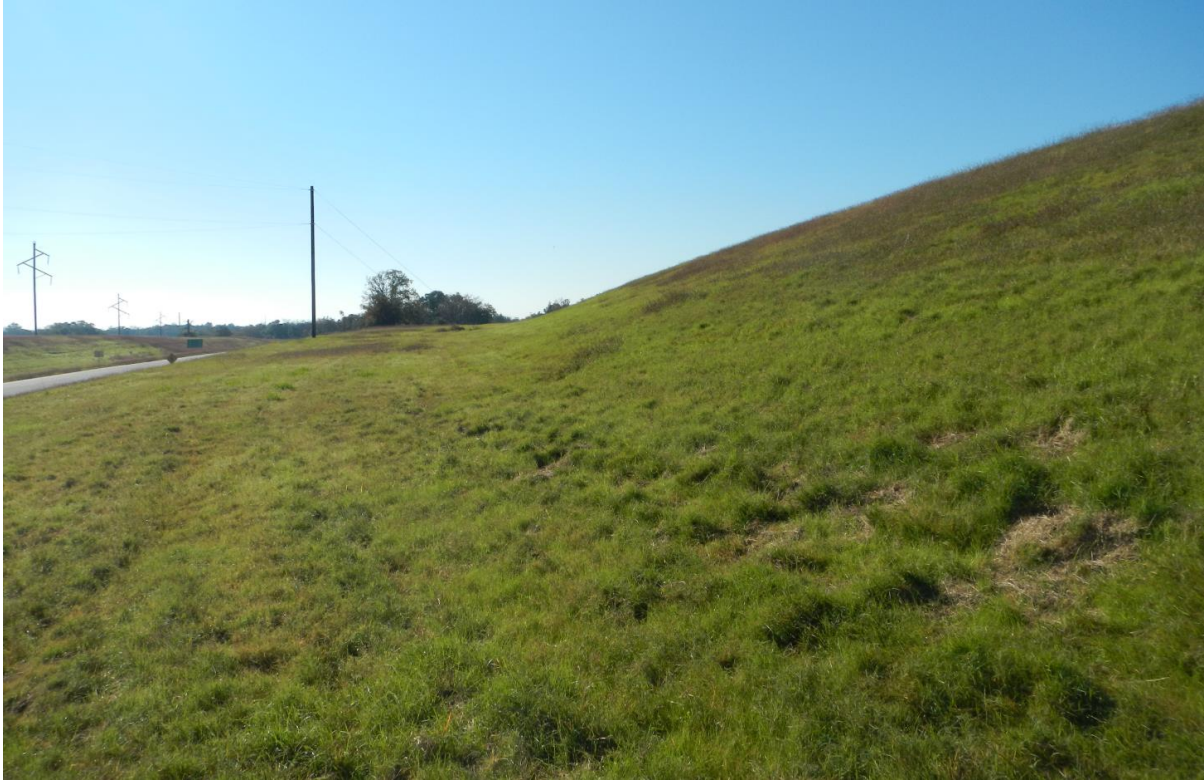
PHOTO 5 – View of East Embankment from Toe Looking South (12-09-2015)
