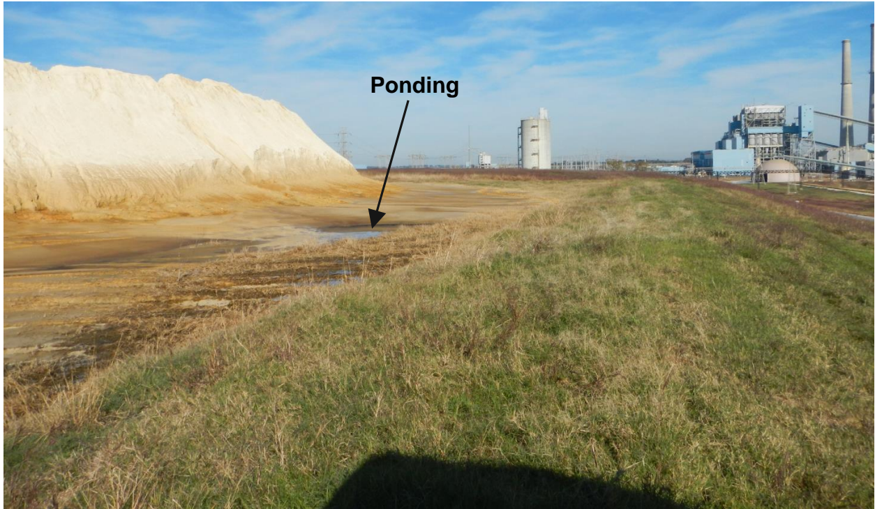
PHOTO 9 – View of East Embankment Crest Looking North (12-09-2015)
