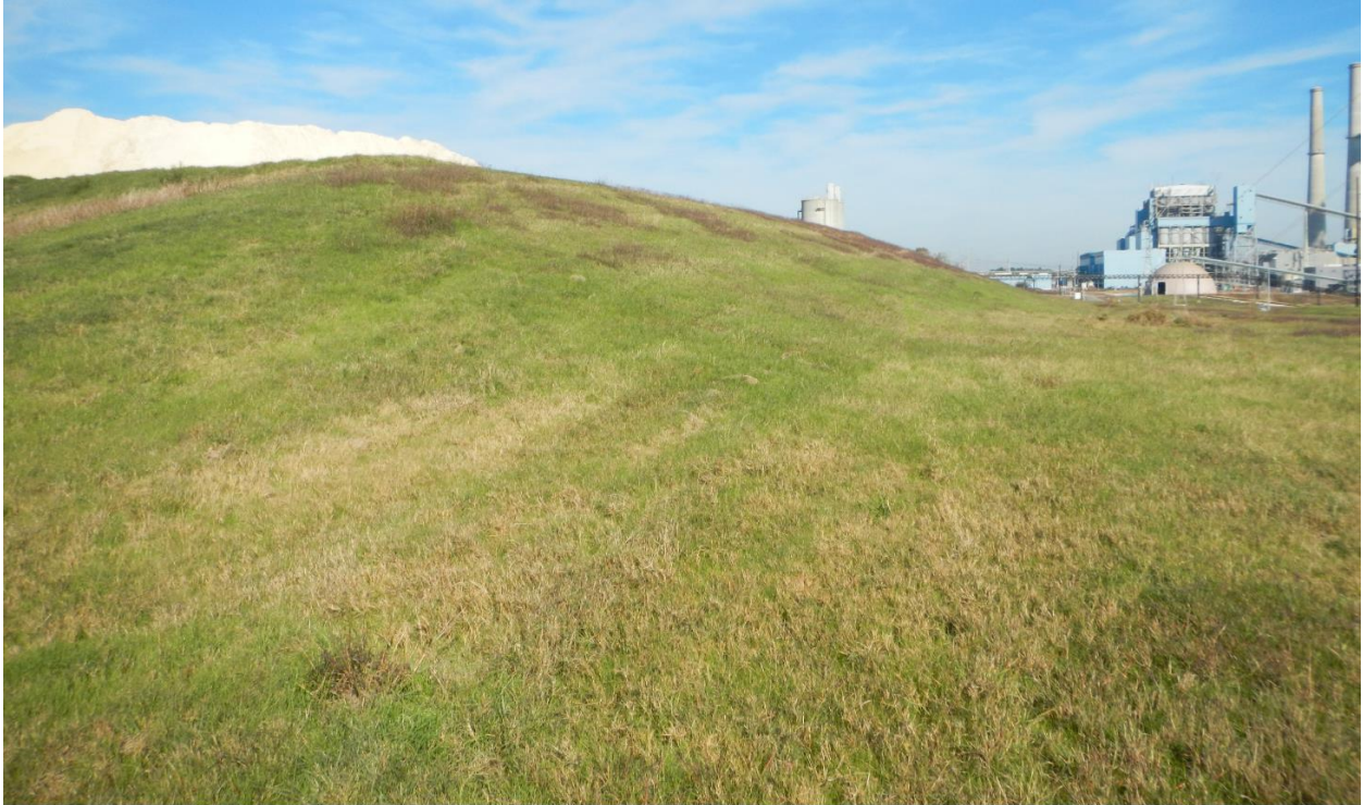
PHOTO 7 – View of East Embankment from Toe Looking North (12-09-2015)
