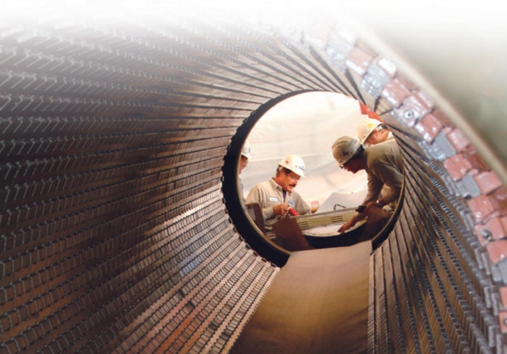
Employees at Sim Gideon Power Plant do maintenance work on the generator shaft of one of the plant's three units.
