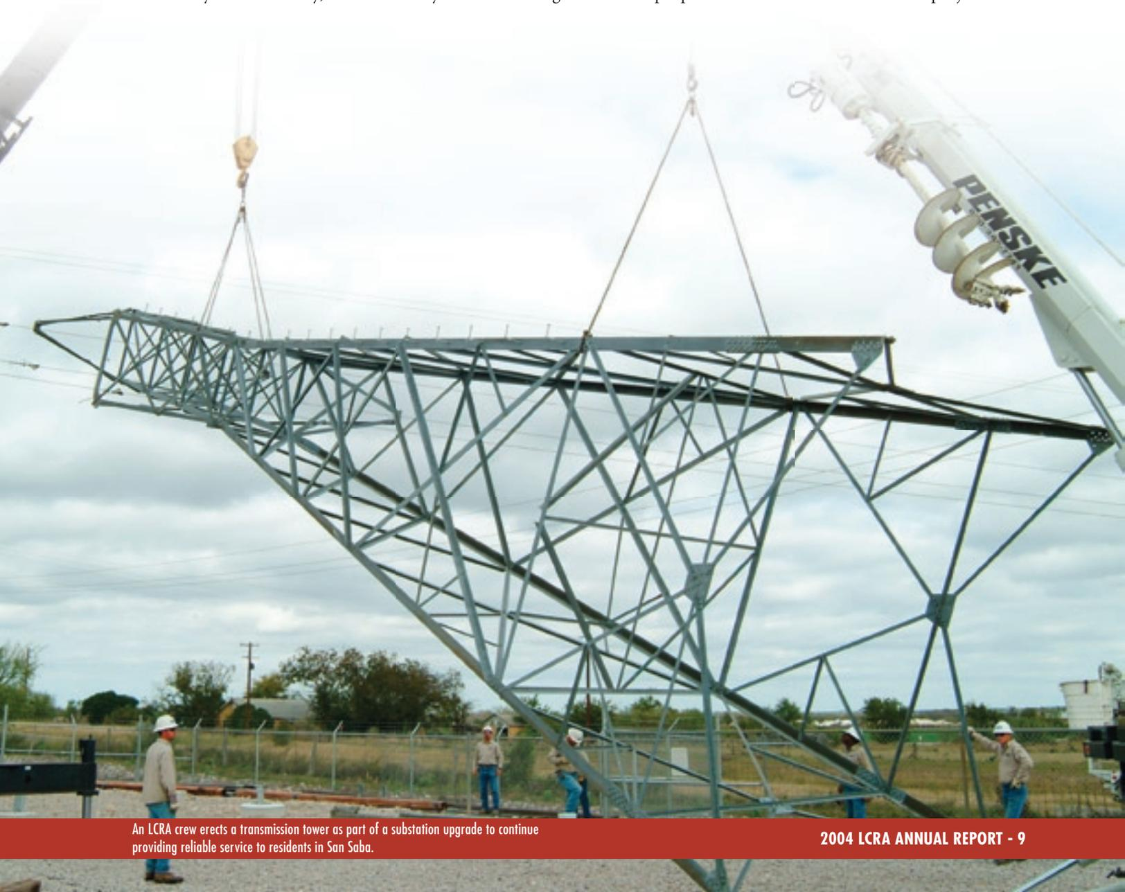
An LCRA crew erects a transmission tower as part of a substation upgrade to continue providing reliable service to residents in San Saba.
